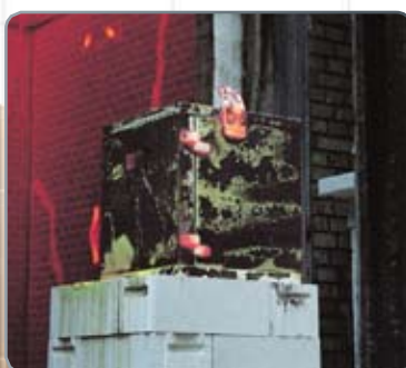
Removal of cabinet from oven
